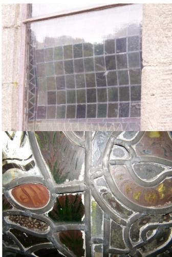
Signs that repair is needed can be any of the following: Windows beginning to bow in or out from the perpendicular; cracks and fissures in the lead (usually alongside solder joints); a rattling sound when windows are gently tapped; glass cracking due to the collapse of the window.
