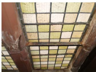
Keep an eye on the condition of supporting bars. If these are very rusty (and especially if such rust is or could be causing damage to surrounding stonework) then they should be replaced with stainless steel bars by a specialist.
